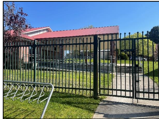
Figure 23. External view from within the primary school facing north towards the hall building.
