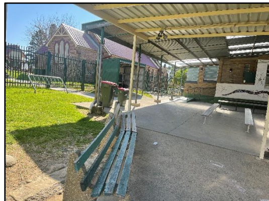
Figure 13. External view from beneath the metal awning over the concrete area, facing north-east towards the St Paul's Roman Catholic Church and the main school building.
