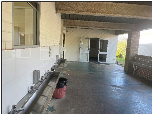
Figure 18. External view to the bubbler area within the southern wing of the main school building.
