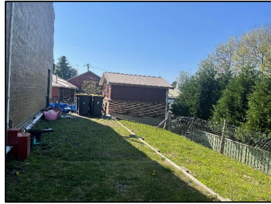
Figure 21. External view to the southern boundary (to the right of the figure) of the school site.
