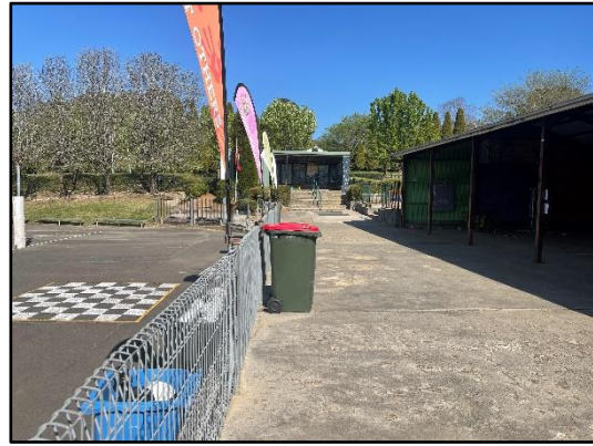
Figure 15. External view from within the school facing west featuring the two weather sheds (both proposed for demolition).
