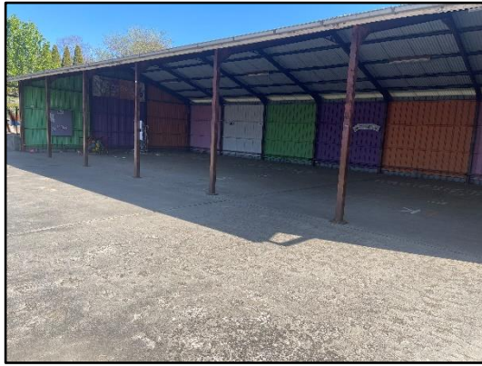
Figure 14. External view from within the school facing north towards the weather shed (proposed for demolition).
