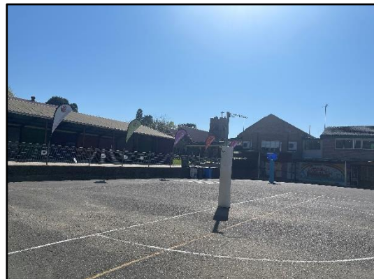
Figure 19. External view from the bitumen area, facing north-east.
