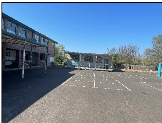
Figure 16. External view from within the bitumen area, facing south towards the demountable (proposed for demolition). The southern wing to the main school building is to the left of the image.
