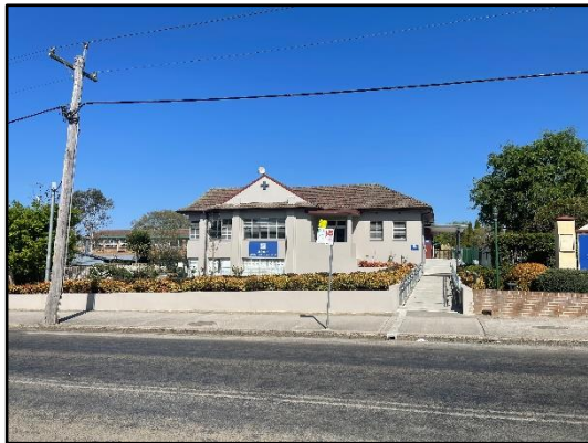
Figure 10. External view from Garrett Street facing west towards the main school building within the St Paul's Primary school.
